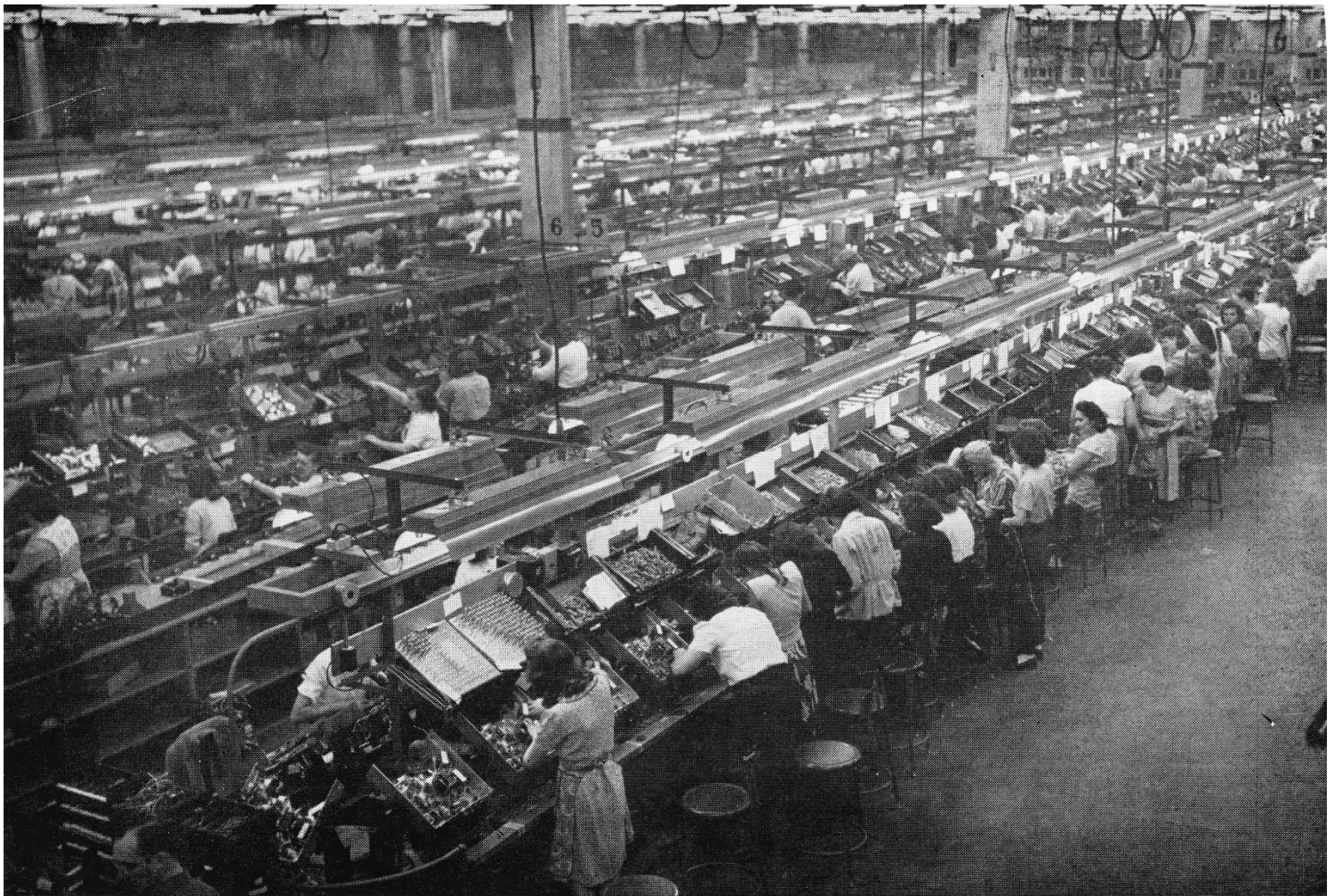
MASS PRODUCTION —General view of manufacturing floor of Receiver Building, with television receiver assembly lines in foreground. By Christmas every line here will be making tele
